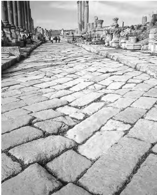
Figure 22.4 Section of a paved Roman road showing curbing and sidewalks, Jerash, Jordan. Photo Andrew Leyerle
